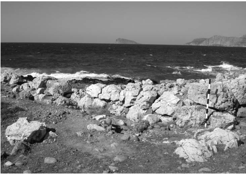
Figure 2. View of the west façade of the ship-shed (Shore House). Photograph by Janet Spiller.
