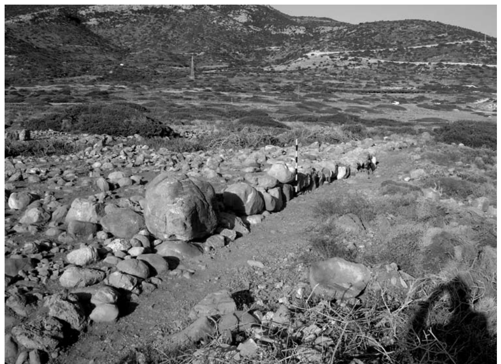
Figure 3. View of wall 5. Photograph by Janet Spiller.
